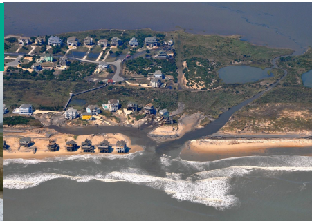
Figure 3. Breach during hurricane Irene
